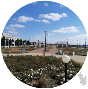
Construction of an embankment along the shore of the Saky Therapeutic Lake, Republic of Crimea, Saki town
