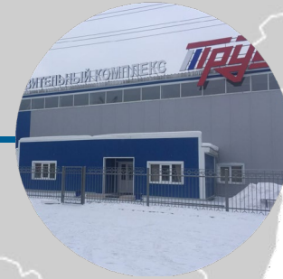
Construction of the "Trud" sports and recreation complex»
