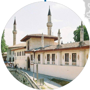
Restoration of the compound of the Khan's Palace facilities
